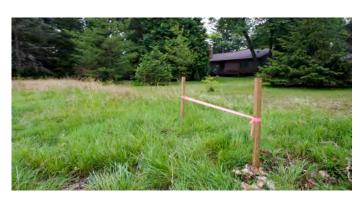
Hanson home are visible just beyond those stakes. The orange tape running between the stakes shows how high the asphalt parking lot slab will be compared to the Hanson property. A reasonable inference from the facts portrayed in Exhibit H1 is that storm water accumulations on the parking lot surface will run downhill onto the Hanson property.
